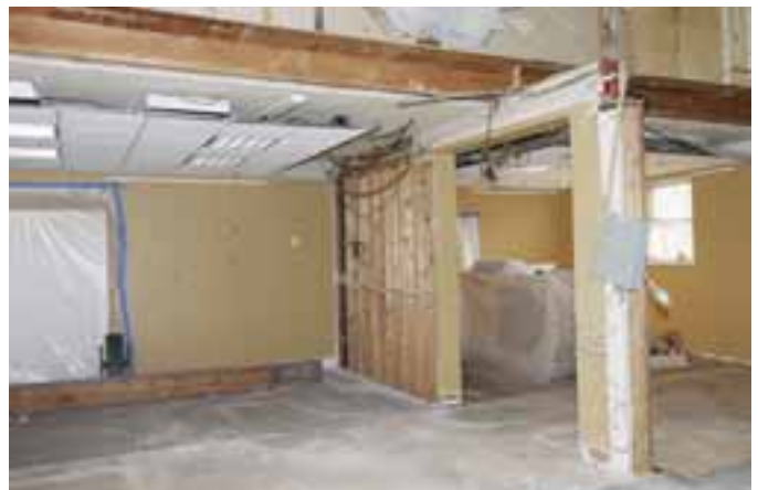
Steel supporting beam to stabilize second floor
