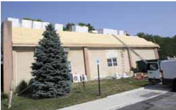
Roof Parking Lot - August 11 Roofing underlayment in preparation for metal roof
